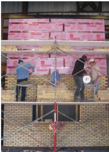
NFPA 285 test wall under construction.
