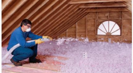
Trapped heat and moisture in the attic can severely jeopardize the performance of a roof. The combination of insulation and a ventilation system helps to keep excessive household moisture and heat out. As a result, the proper conditions and temperature are better maintained in the attic and on the roof deck throughout the year.
